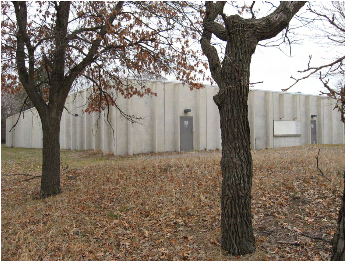
The new concrete building that replaced our burned-out original indoor range. The white rectangle is the outside opening for concessions. (viewed from the southwest)
